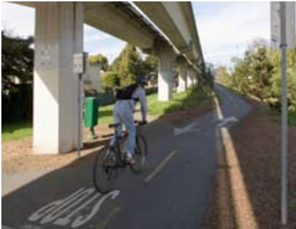
Class I Bikeway (Bike Path) Provides a completely separated right of way for the exclusive use of bicycles and pedestrians with crossflow of motorists minimized.
