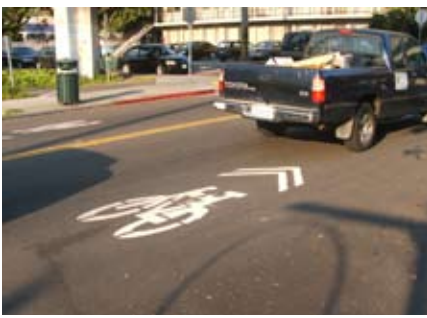
Class III Bikeway (Bike Route) Provides for shared-use with pedestrian or motor vehicle traffic.
