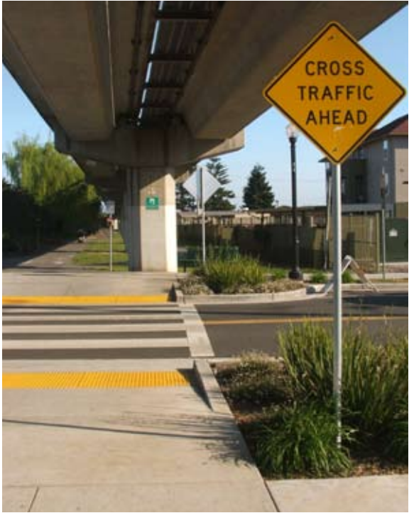
Visible crosswalks like this one on the Ohlone Greenway are important for safety along the Greenway route.
