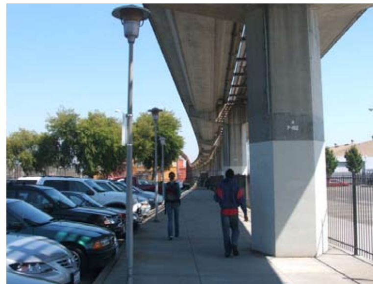
Sidewalk underneath BART tracks in BART parking lot
