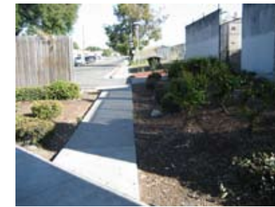
Widen this connection between Bay Fair BART and Elgin to provide space for cyclists
