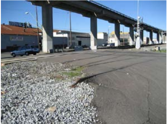
Existing condition of the railroad crossings
