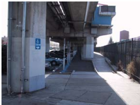
Signage and a wider pathway are needed at the Hayward BART entrance from B Street
