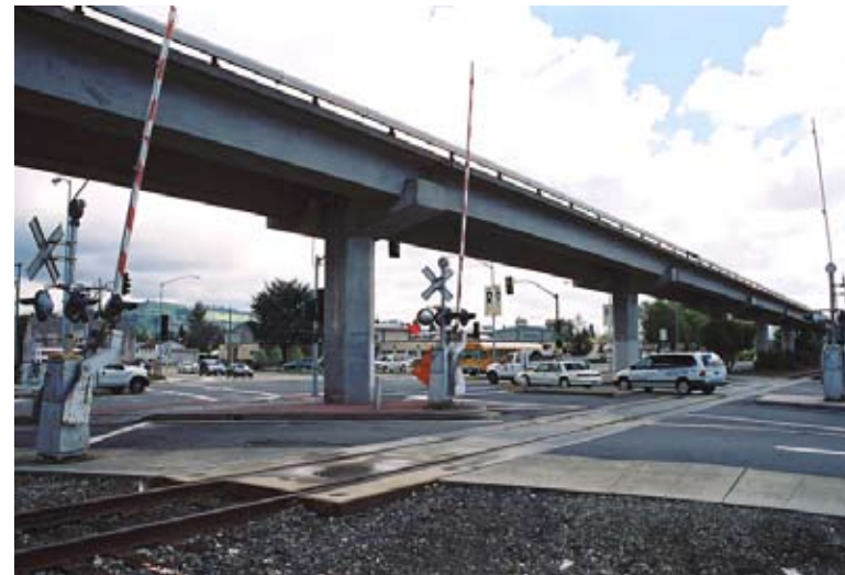
The Marina Boulevard and San Leandro Boulevard intersection
